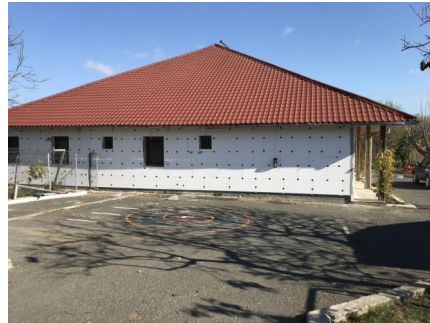
In the spring, the walls will be rendered with plaster and painted to withstand harsh weather.
