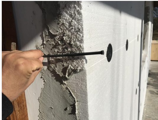
Strengthening struts are fitted to each sheet of insulation.
