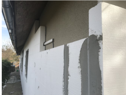
Insulating sheets 5cm thick (2 inches) are glued to the existing walls.
